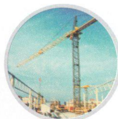
Cantiere Building site
